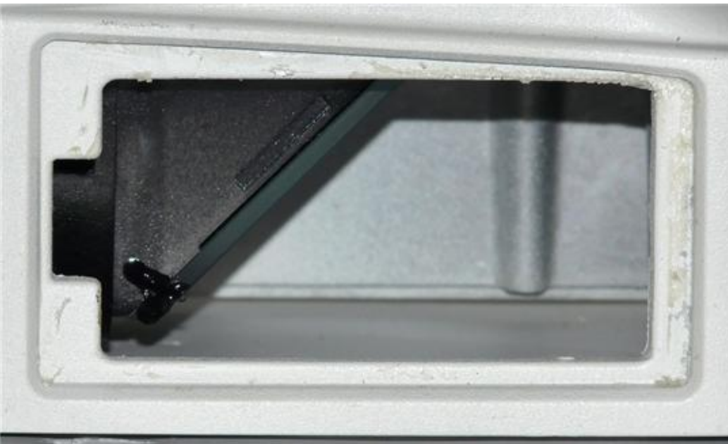
(2): Ready to install new plate.
